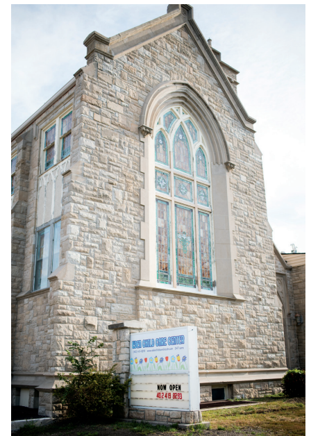
Historic stained-glass windows still need restoration at 2980 Holdrege Street.
